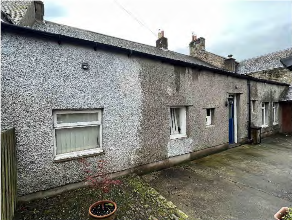
Figure 1: Rear of property
